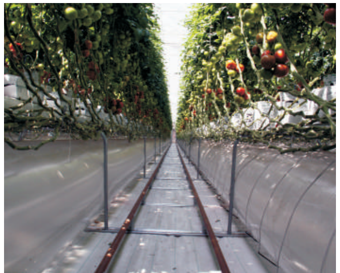
Pressure controlled air distribution under the crop
