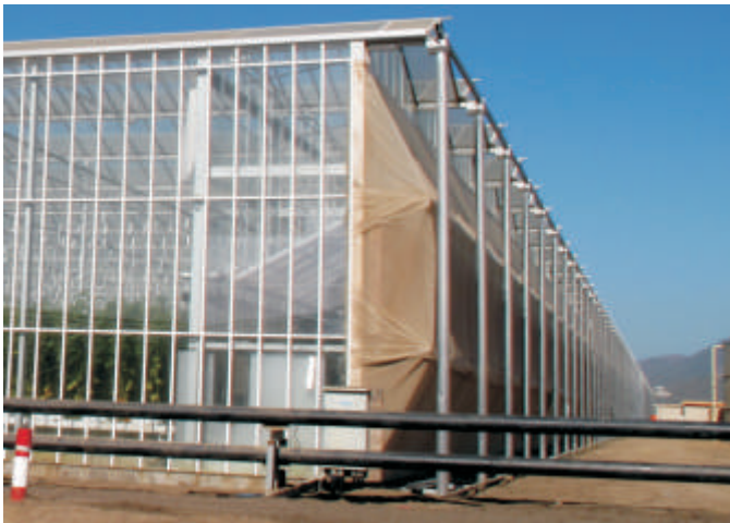
Air intake insect screening along the entire gable end. The air mixing chamber is located just inside the gable end.
