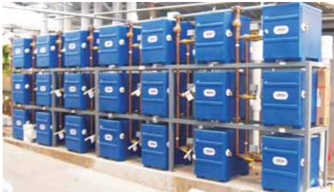
Multi-Boiler System Photo Courtesy TrueLeaf Technologies
